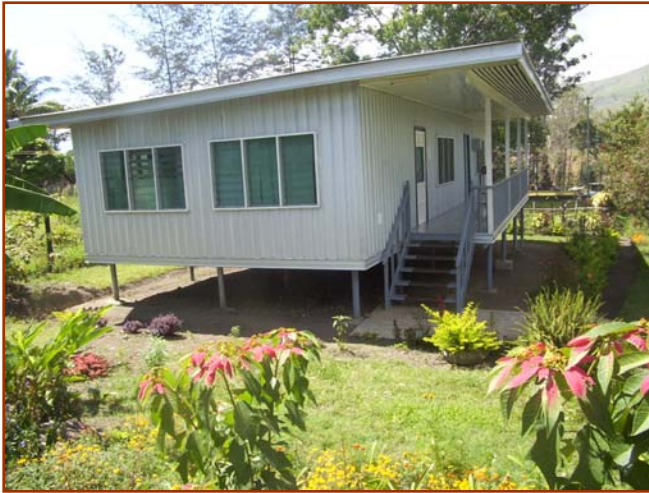
Picture two. Kapakamaliki Sub-health Center building. This is run by Four Square Mission
